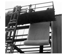
sounds within the building. Canadian Metal Building Insulation provides thermal efficiency, helping to keep heat inside the building in winter and outside in summer. When faced with a vapour retarder it helps control condensation on the inside surfaces of the building's roof and walls.
