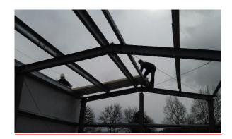
3. Use roof layout plan to continue installing proper panel in locations moving along the roof line.
