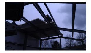
4. The tape tab should be pulled as you move forward on the roof. Tape tabs should not be left unsecured for more than a few minutes (Dust and jobsite conditions can affect the adhesive on the tape the longer it is exposed).
