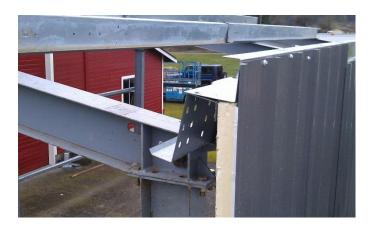
2. A light gauge ridge pan should be installed between the two ridge purlins so that there is a place for the roof panels to sit on where they meet at the ridge.
