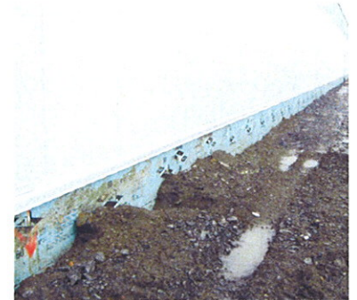
Fasten Extruded Polystyrene on to concrete foundation wall.
