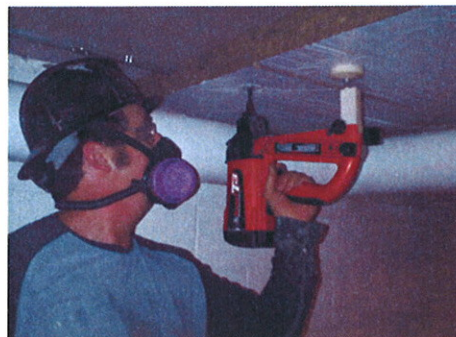
Fasten Laminated Roxul Board onto concrete ceiling in parking garages with ease.
