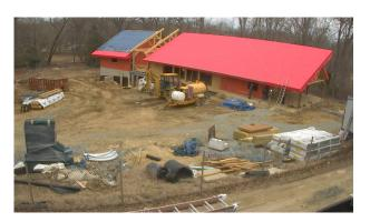
Over 4,600 sq. ft. of SlopeShield SA Self-Adhered Water Resistive Roof Underlayment Sheet (red) was installed on the Alice Ferguson Foundation's Potomac Watershed Study Center. The Potomac Watershed Study Center marks one of several VaproShield projects seeking Living Building Challenge certification. All photos courtesy of TrueLook Webcams.
