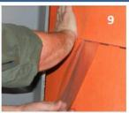
Use the opposite hand to smooth the Smooth out wrinkles with hand pressure. two layers together as the release paper is removed.
