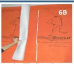
Apply Dow 758 or Tremco Butyl sealant in a single bead down the membrane to the bottom of the
