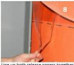
Line up both release papers together so they can be pulled down the wall with one hand.
